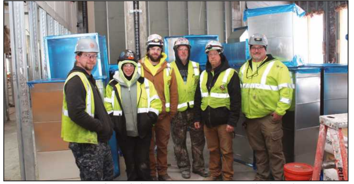
WITH A WIDE VARIETY OF DUCTS providing a backdrop on the 18th floor of the Residences @ 150 Bagley building in Detroit, we asked this group of Sheet Metal Workers Local 80 members coming off their break to pose for a photo. They include (l-r) Robert Schell, Shannon Nelson, Brandon Struck, Ryan Pabst, Dan Quinn, Sr. and Eric Allen. They're employed by Sylvan, Inc.
