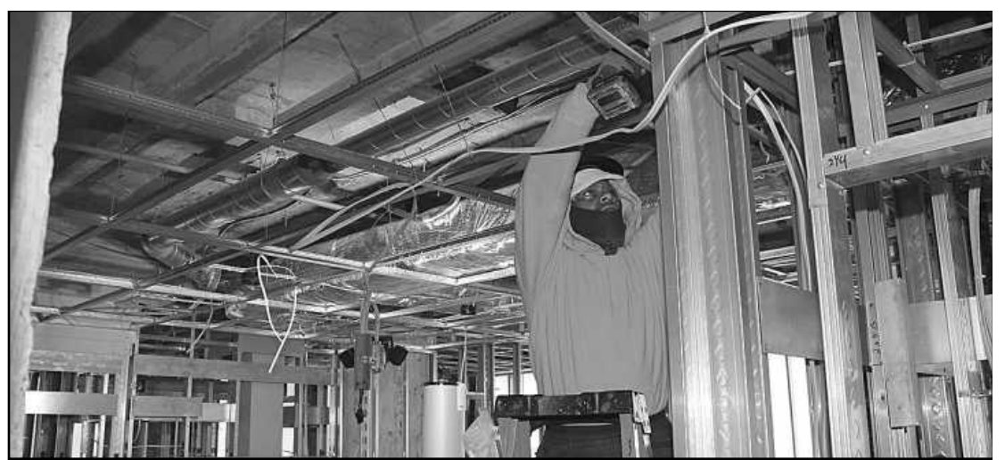
SETTING A STRAP at the Residences @150 Bagley project in Detroit is Kennan Kidd of IBEW Local 58. He's employed by Edgewood Electric.
