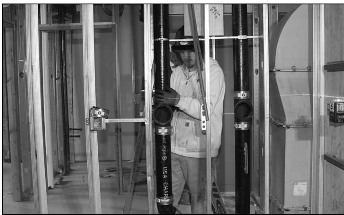
SETTING A FOUR-INCH cast iron drain pipe on the sixth floor at the Residences @ 150 Bagley project in Detroit is Earl Ray of Plumbers Local 98. He's employed by Ben Washington and Sons Plumbing and Heating.
